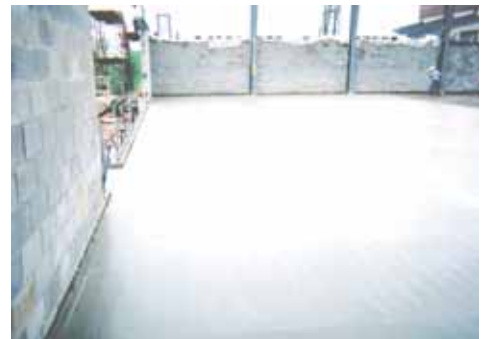
Mapleton High School gym floor
