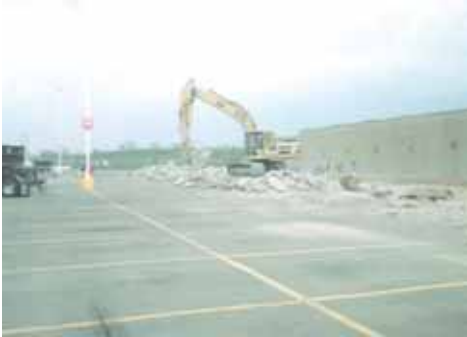
Meijer Store addition & garden center
