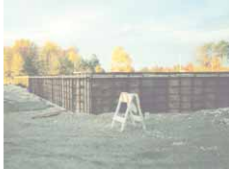
12,000 sq. ft. steel building foundation & piers
